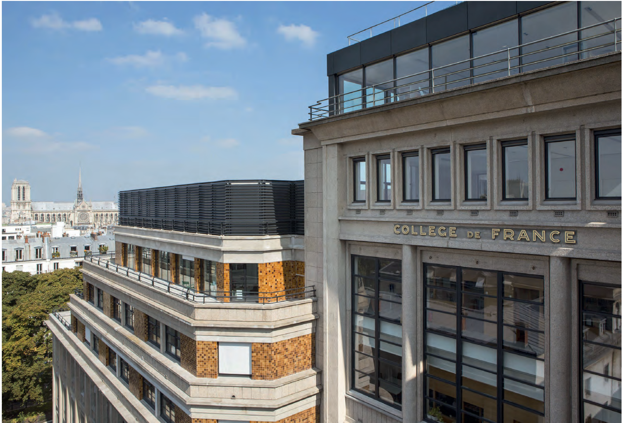
Rooftop terraces at the Marcelin Berthelot site.
